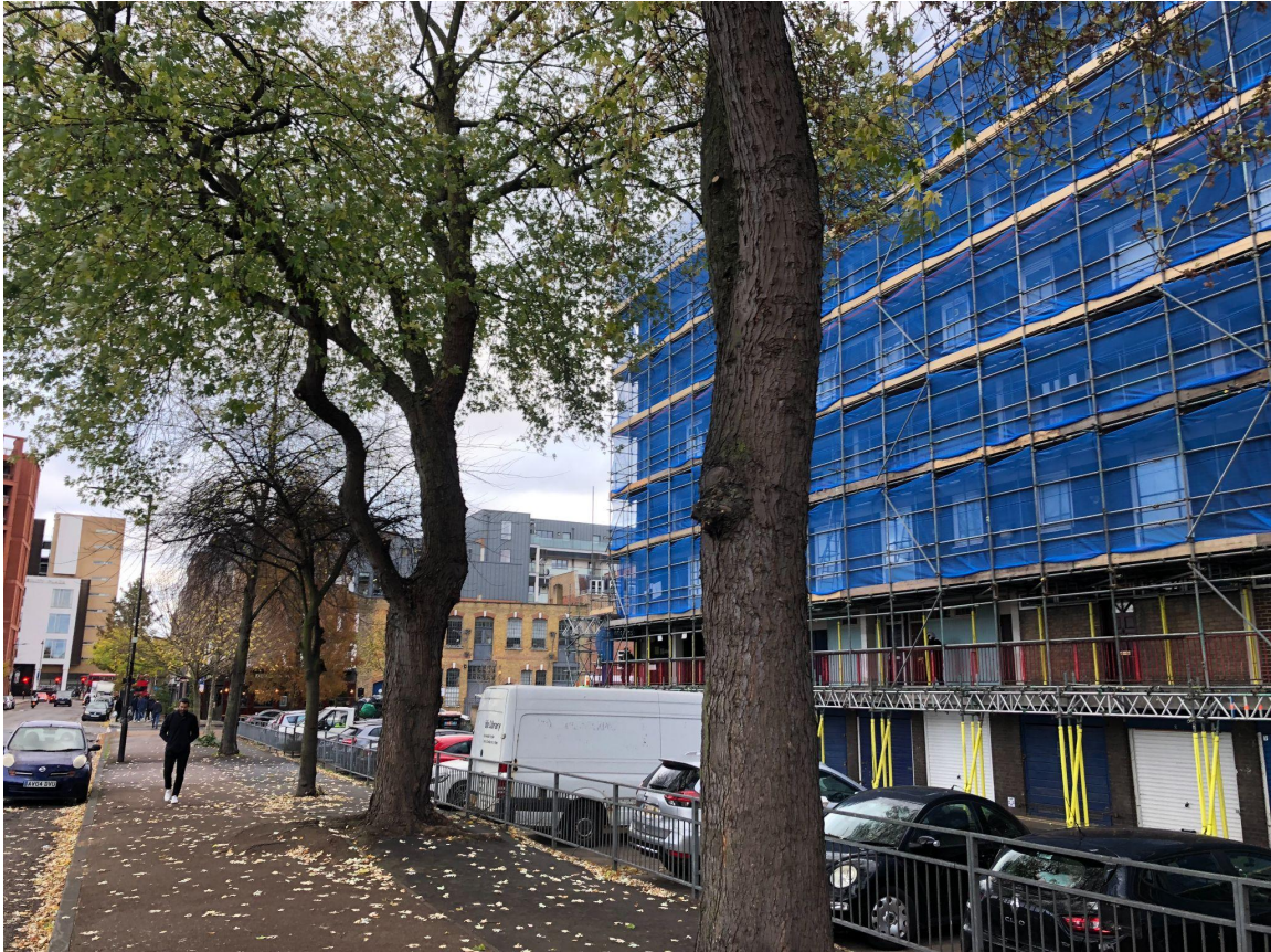
Looking west down Downham Road towards Hertford Road site:
