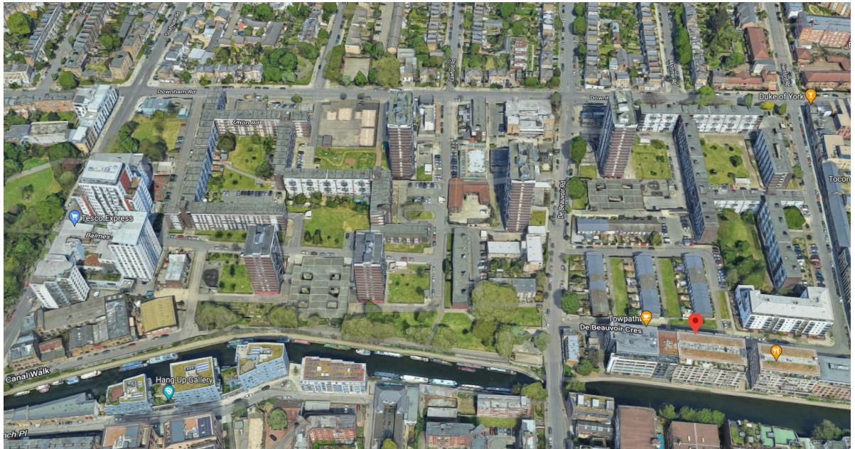
The estate, looking north.
